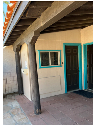
Exterior T1-11 storage room to be demolished
