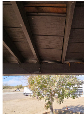
Failed decking replaced with T1-11 siding
