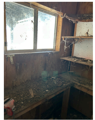
Interior of storage room to be demolished
