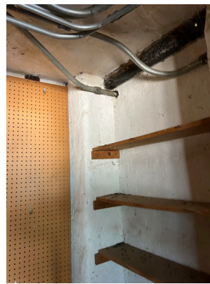
Interior of storage room to remain
