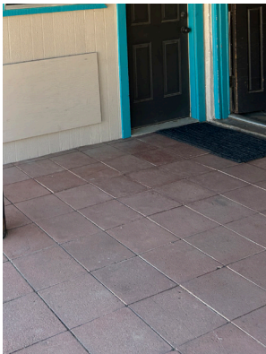
Floor tile to be salvaged
