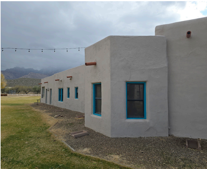
North elevation looking east
