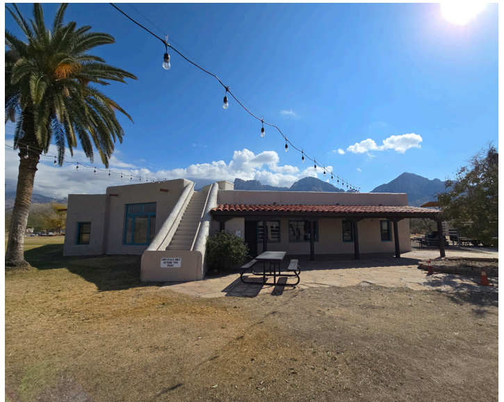
North elevation looking west
