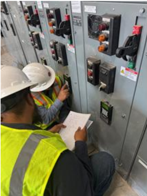
La Cañada Booster Motor Control Center panel programming (left) Water Control Systems staff programming La Canada Booster Station new PLC (right)
