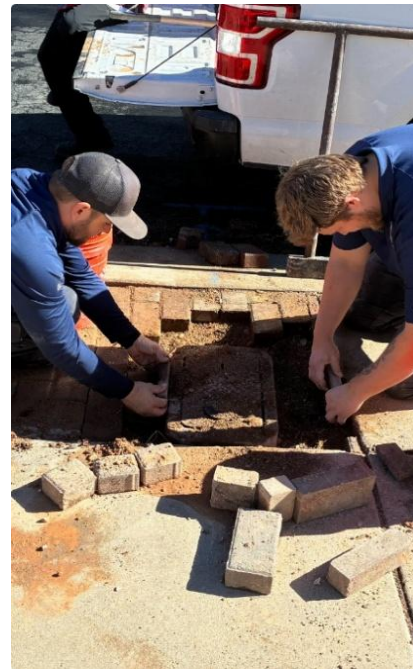
Meter Operations staff drilling our meter lid to install transponder (left). Meter Operations staff replacing pavers around meter box after repairs (right).
