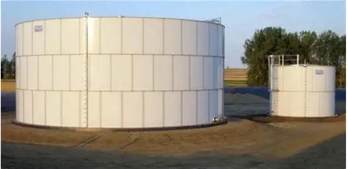
The photo above shows an illustration of what our temporary tank would look like at site during tank rehabilitation
