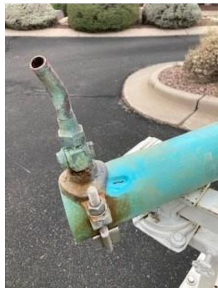
Water Distribution staff dug up a 4" main on Alder Springs Pl. (left) to repair a bad saddle tap (right)
