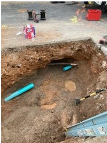
Water Distribution staff dug up a 4" main on Alder Springs Pl. (left) to repair a bad saddle tap (right)
