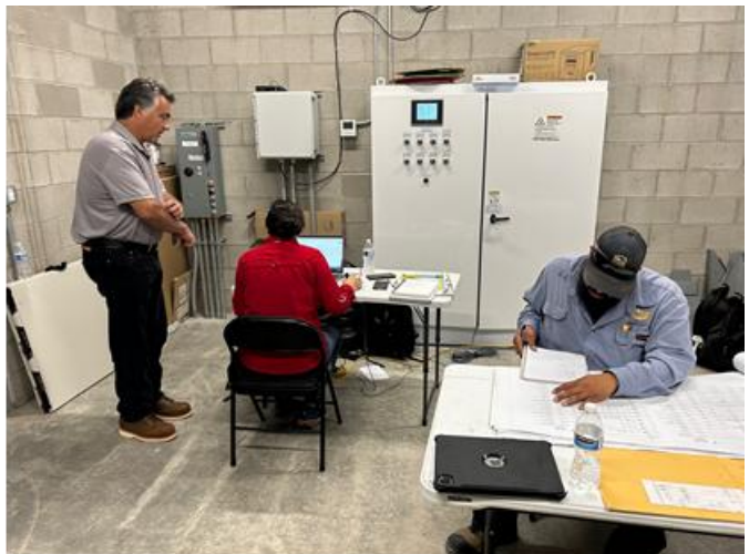
La Cañada Booster Motor Control Center panel programming (left) Water Control Systems staff programming La Canada Booster Station new PLC (right)
