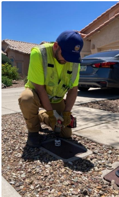
Meter Operations staff drilling our meter lid to install transponder (left). Meter Operations staff replacing pavers around meter box after repairs (right).
