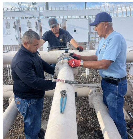
Staff replacing a broken check valve at a booster site (right).
