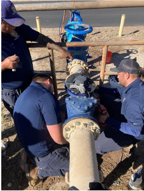
Meter Operations staff replacing a 6" meter for La Cholla Airpark (left). New Meter Operations staff training in the field (right).
