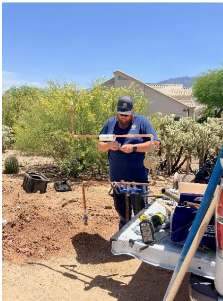
Staff repairing and testing Town of Oro Valley backflow prevention assemblies (left and right)
