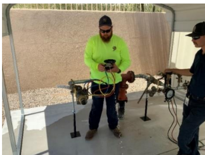
Staff collecting compliance water samples (right). Staff repairing and testing Town of Oro Valley backflow prevention assembly (left).
