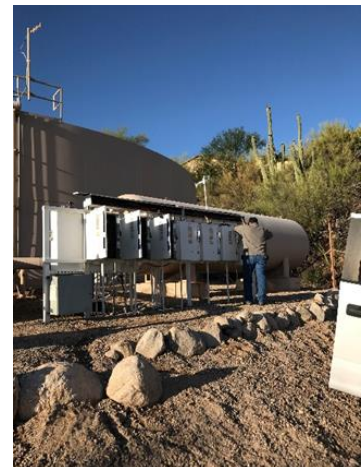
Water Control Systems staff calibrating and programming new instrumentation (left). Water Control System staff performing preventative maintenance on electrical controls (right).
