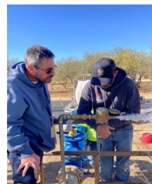
Meter Operations and Water Distribution staff repairing a damaged AMS (left).
