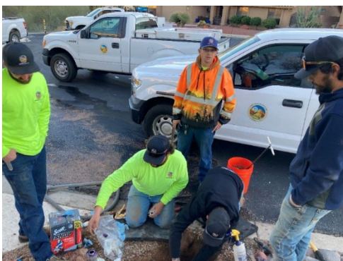
Meter Operations and Water Distribution staff repairing a damaged AMS (left).
