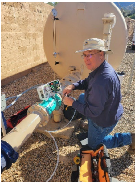
Water Control Systems staff calibrating and programming new instrumentation (left).
