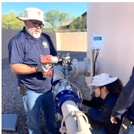
Staff installing a flowmeter at Glover Reservoir (left). Staff replacing a check valve on a booster pump discharge at Vistoso Reclaimed Plant (right).
