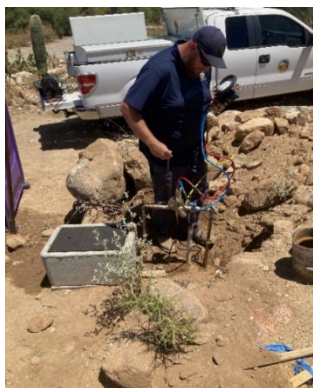
Staff repairing and testing Town of Oro Valley backflow prevention assembly. (left).
