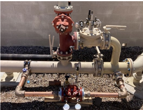
The Utility's Water distribution staff installed a new 2" bypass PRV at Lambert booster station to assist with pressure sustaining in the surrounding neighborhood.
