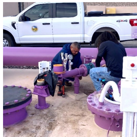
Staff installing a flowmeter at Glover Reservoir (left). Staff replacing a check valve on a booster pump discharge at Vistoso Reclaimed Plant (right).
