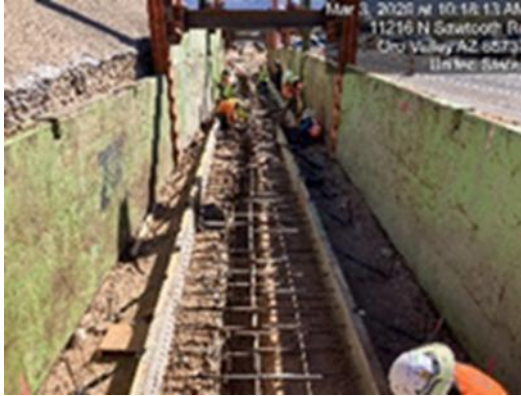
Inspecting reinforcing steel and forming on retaining wall 1.
