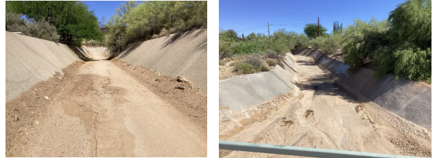
Vista Del Oro Wash – after photos
