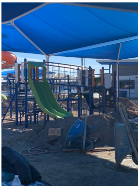
JDK Playground Renovation
