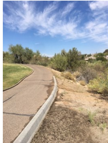
Curb clean up—after
