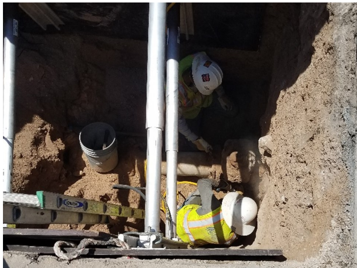
Water utility staff replace a faulty buried water valve.
