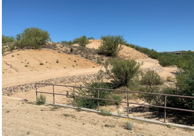
The access road and slope stabilization riprap work is completed for the Nakoma Sky well site
