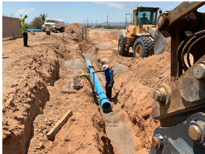
Hunter Contracting installs a section of 12-inch PVC water pipe
