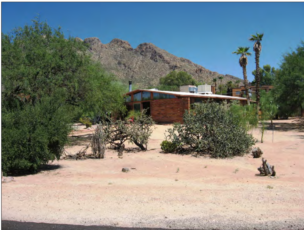
Figure 33. Ranch-style residence built in 1959 in Shadow Mountain Estates (2009).
