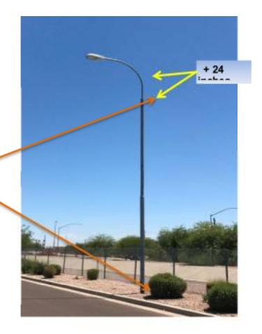
The Top and Bottom Points on a Telescopic Streetlight Pole to Calculate the Vertical Height of the Existing Streetlight Pole PLUS
