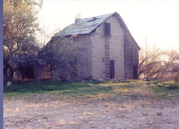
Steam Pump Building
