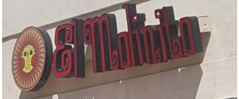
10180 North Oracle Road (adjoining parking lot with San Jose Plaza) Illuminated Pan Channel Letters, raceway-mounted
