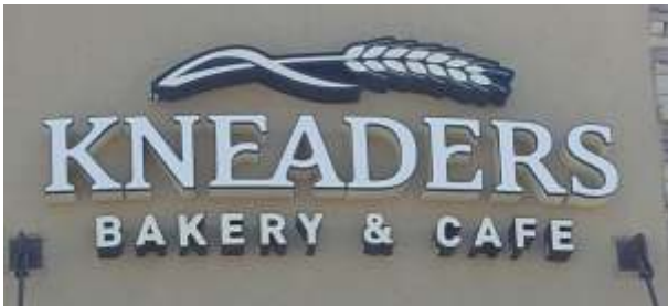
9660 North Oracle Road Illuminated Pan Channel Letters, surface-mounted with accent pill cabinet
