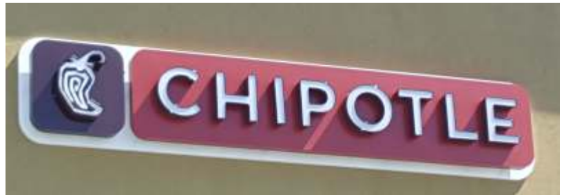
10604 North Oracle Road Illuminated Pan Channel Letters, raceway-mounted with accent pill cabinet
