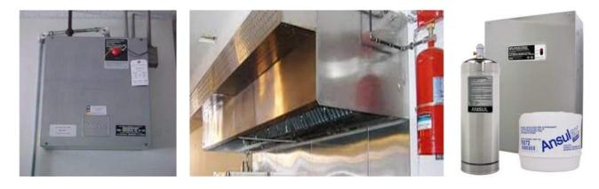
Kitchen hood extinguishing systems shall be installed in accordance with the International Fire Code (IFC), the International Mechanical Code (IMC), applicable National Fire Protection Association (NFPA) standards and the manufacturer's recommendations. The installing contractor shall perform all tests.
