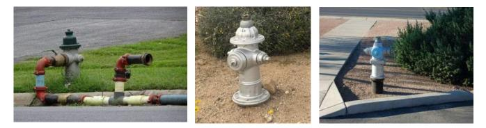
Fire hydrants shall be in place and operational prior to combustible construction materials being brought onto the site. Operational is defined as being fully tested, chlorinated, and approved by the water department and GRFD. A hydrant shall be located within 150 feet of stored combustible construction materials. Additional hydrants shall be installed in accordance with the Town of Oro Valley/Marana or Pima/Pinal County requirements.
