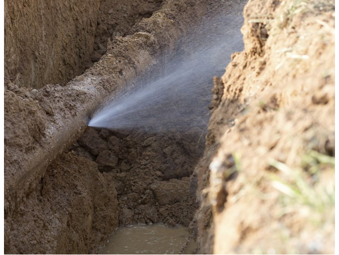
Buried distribution main leaks are a common contributor to lost and unaccounted for water.
