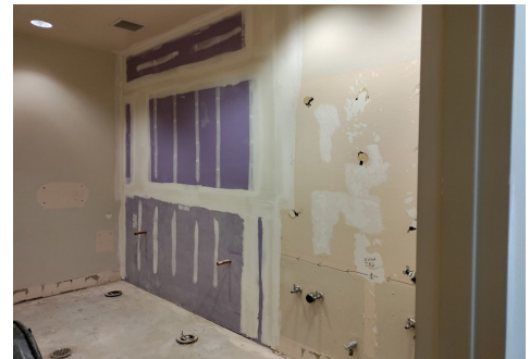
OVPD Main Station lobby restroom construction
