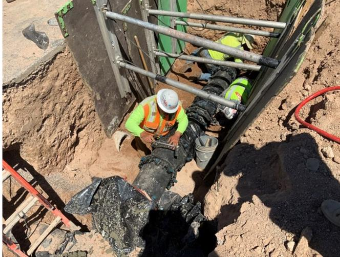
*Pictured above the contractor installs a section of 12-inch ductile iron water pipe.*
