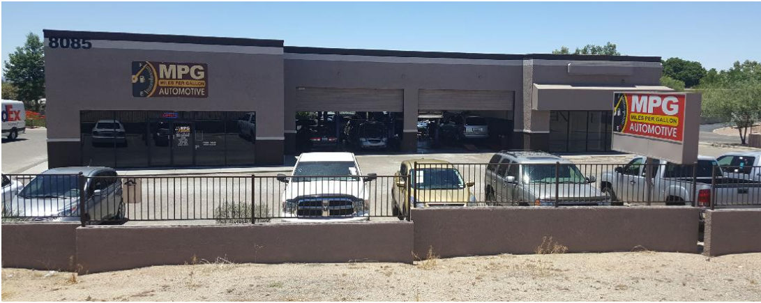
Existing East Elevation (front of building)
