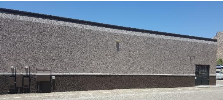
Existing South Elevation (side of building)
